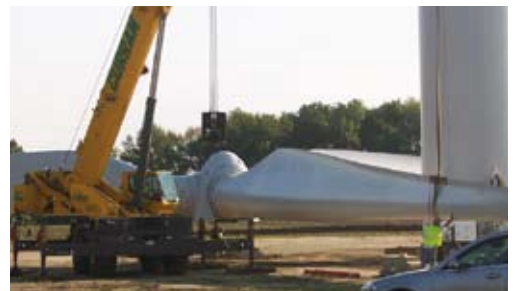
Grove RTC890E on site at the Noble Thumb Wind Park Phase
